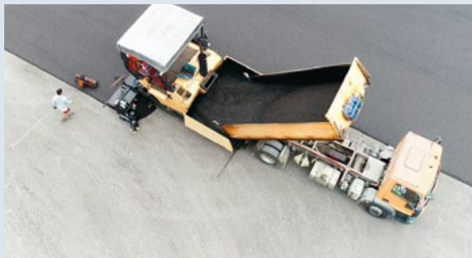
3. CONSTRUCTION: Polytan lays an elastic underfloor made of rubber granulate and a CO 2 -based binder on a hockey pitch in Krefeld.
